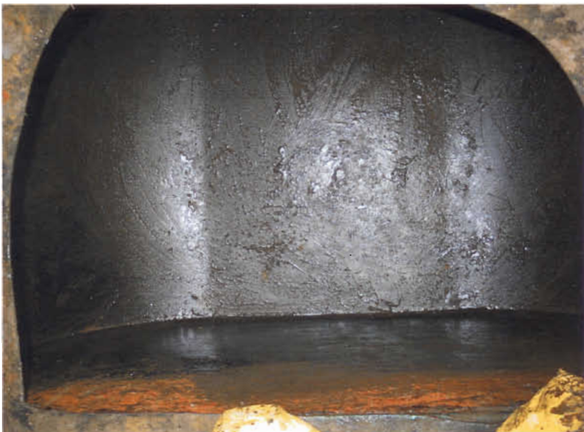
Figure 2: Tank interior end furthest from 34th Avenue, after cleaning
