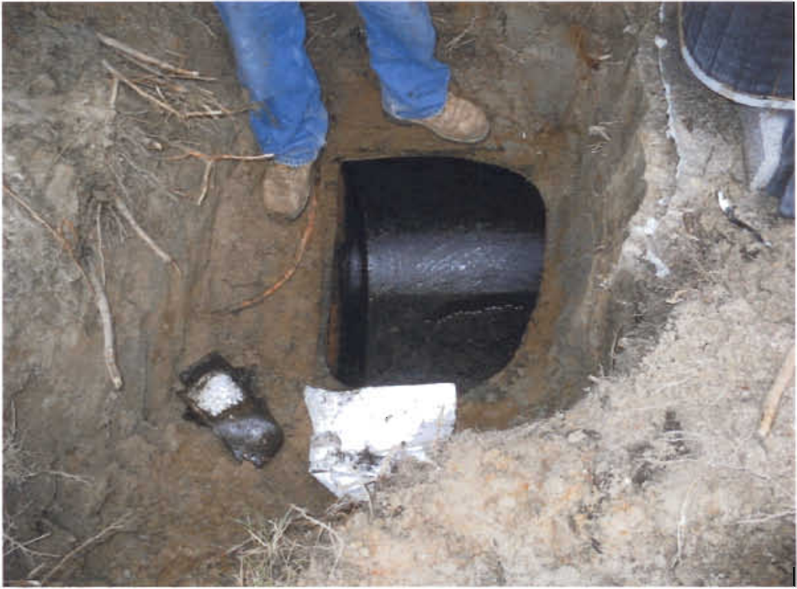
Figure 4: Tank excavation relative to the air conditioner
